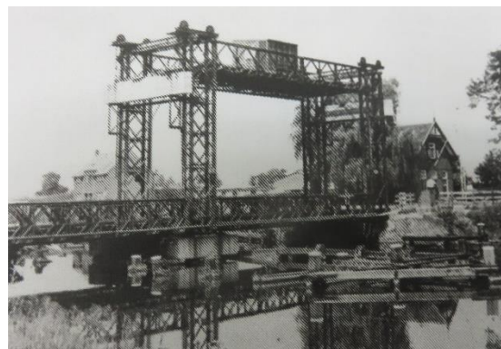
Class 70 Bascule Bailey Bridge being raised
