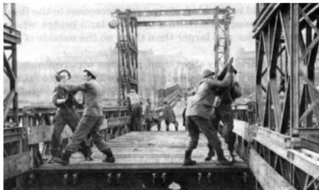
Class 70 Bascule Bailey Bridge being raised
